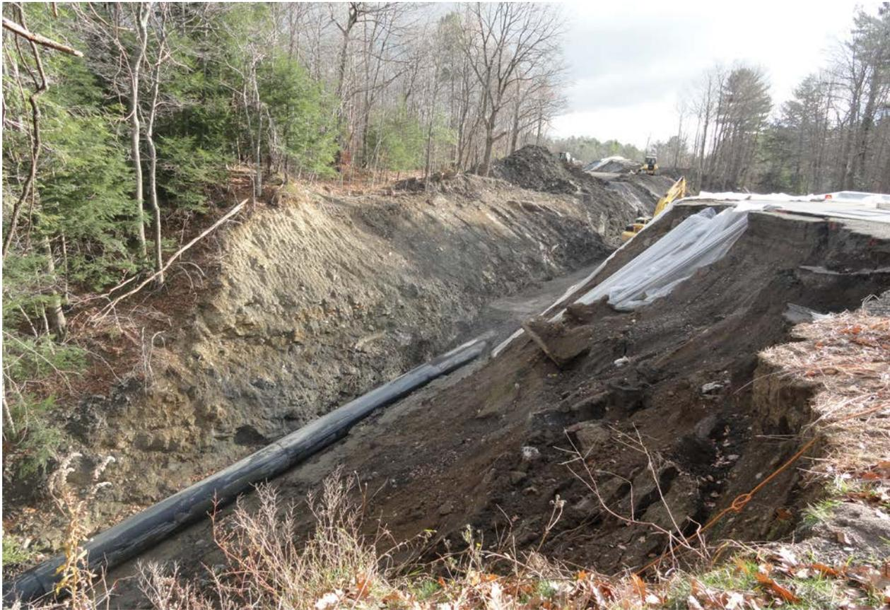
Italy Turnpike culvert failure & landslide -- new culvert installed, backfill in progress
