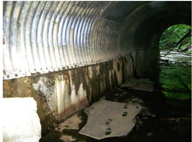
Broken, spalled concrete at north support wall
